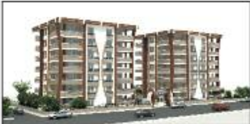
ALTUNDAL İNŞAAT - KINEBA PARK
