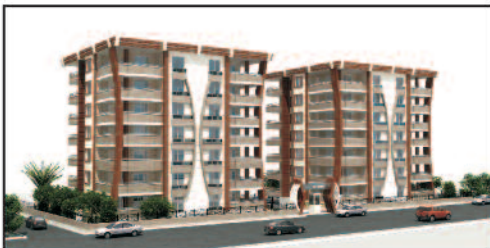
ALTUNDAL İNŞAAT - KİNEBA PARK
